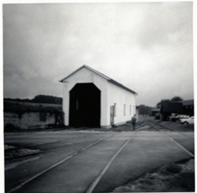
This is the working engine house, and that's the man I mentioned who lined the inbound train up. The track trailing off to the right is a leg of the wye; the track in the left foreground runs into the old engine house. I took a picture, but there isn't much there. The remains of Plymouth no. 8 were inside.
