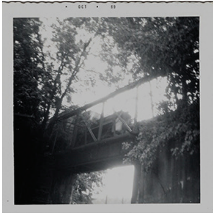
I didn't have much time to set this photo up, and it was raining. But this is the famous iron bridge near Tolna. (The iron work still had a builder's plate dated in the 1870's, before the RR was built. Prolly moved here from elsewhere. The iron work supports its own weight; the deck long ago was replaced by steel girders.)
