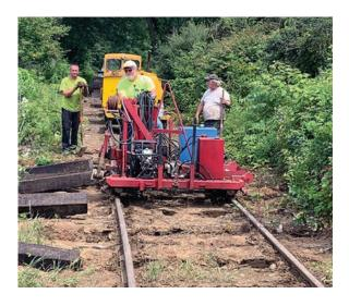
On Sunday, we replaced a broken joint bar east of MP6, replaced numerous loose track bolts, dug out another culvert (by hand), and slushed 17 ties down by the old pumpkin patch.
