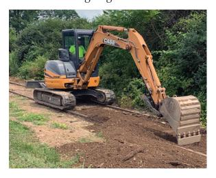
Mike Ruane ran the tie inserter. As you can see the track is in poor condition here with dirt and no ballast and all of the ties are rotten with no spikes holding the rail.
