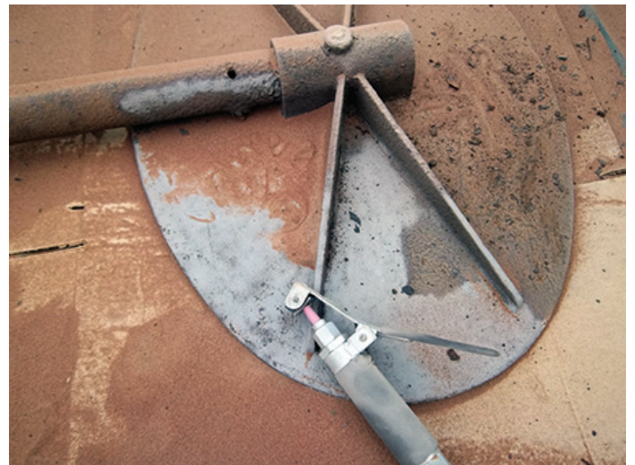
Sand blasting of back of "W" sign. Note another bullet hole on upper pole
