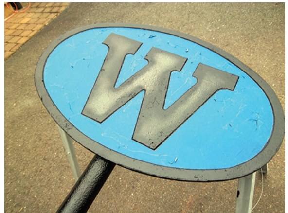
Sign taped off for application of white paint
