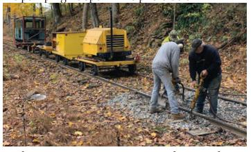
We have more tamping to do on this stretch and will be scheduling that to be done on Friday Dec 3rd if the ground is not frozen. Installing ties can be tricky. The tie needs to be at the right height in the crib. Too high and there is a hump in the track, too low and there is a dip. Dips accumulate water and allow ties to pump up and down, giving a rough train ride with potential for broken rails. There is also spot tie work to do between the cis-
