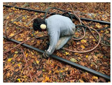
We raised two swales and ballasted and tamped a spot where the ties were pumping mud causing the train to go up and down. Chris Lutz, John Pope and Jim Tapley are using the air tampers at the pumping tie spot in the photo below.
