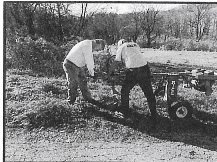
One of the benefits of being a volunteer with the Friends of the Stewartstown Railroad is the opportunity to work with all types of equipment. Here our volunteers are preparing to use a power-auger to open a post hole for a crossbuck to be installed at the intersection of Tolna Road and Elm Drive. Photo by Miles Weaver.
