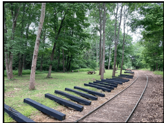
New ties donated by Koppers Inc. awaiting insertion near the picnic grove.
