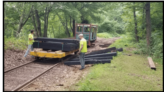
Some of the recently donated ties from Koppers Inc. being unloaded at the worksite.
