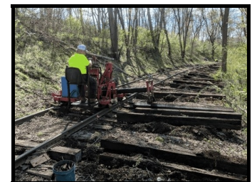
The tie inserter at work! Photo by Miles Weaver.
