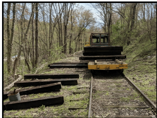
Staging crossties at one of the many worksites along the Stewartstown Railroad. Photo by Miles Weaver.
