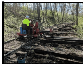
The tie inserter at work! Photo by Miles Weaver.
