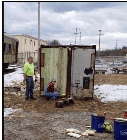
Building a new door for the Friends' storage container.
