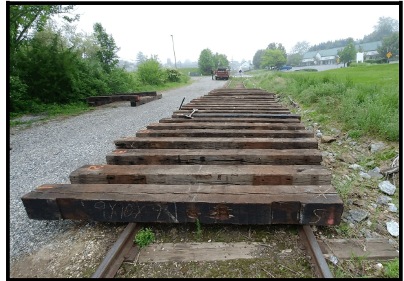
Yes, these are railroad ties on top of the rails! They are being sorted by size for installation on the Stewartstown Railroad's iron bridge. Photo by John Nolan.
