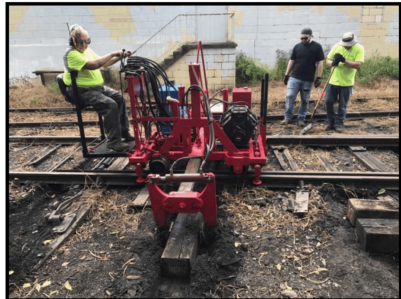
Tie inserter in action on the westend trackage.
