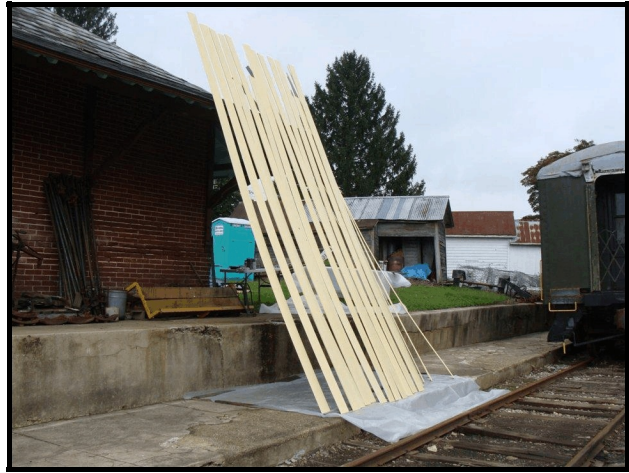
New cedar siding ready for installation on the upper floor of the station in Stewartstown.
