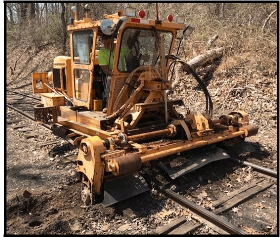
The Stewartstown Railroad's scarifier preparing a section of track for tie replacement.
